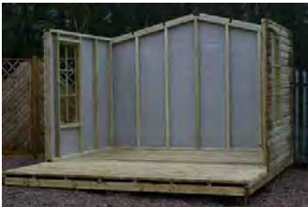
Step 9 - The same is repeated for the other side panels, screwing together the panels as you go.
