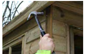
Step 20 - Corner fillets are provided and attached to each corner. This covers the exposed panel edges.
