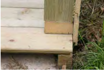
Step 5 - The side panels sit on top of the floor panel. The cladding over hangs the floor panel and finishes flush to the edge.
