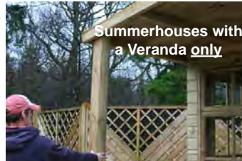
Step 15 - Two support posts are supplied that sit within framework of roof overhang to front of building.
