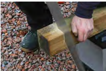
Step 17 - Use a handsaw to trim off the excess post, make sure to only cut off the flat end of the post.
