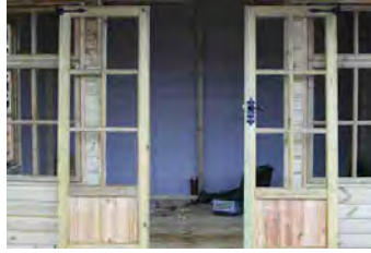
Step 28 - Position the doors on 10mm packers, allowing an equal clearance on each end and between the doors.
