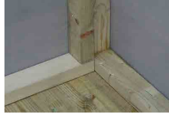
Step 7 - The shed frame should butt together tight in the corners.
