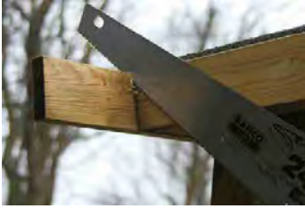
Step 27 - The access front and rear edging boards are trimmed with a handsaw for a perfect fit.
