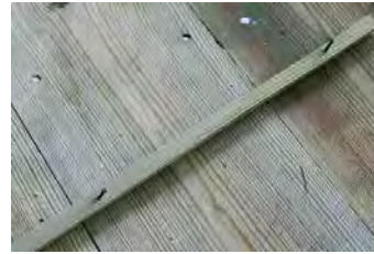
Step 37 - Prime the window beading using the glazing pins provided. (Tap nails into position along length of bead.)
