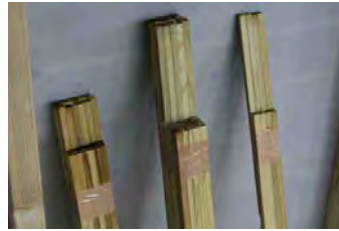
Step 36 - Three small packs of timber have been supplied that are marked for further use e.g. windows & door frames.
