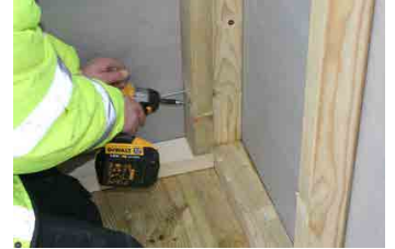
Step 8 - The panels are screwed together through the framework.
