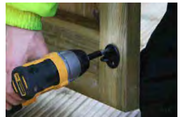
Step 34 - Fit the keep element onto the door at the same height for ease of securing doors in open position when needed.
