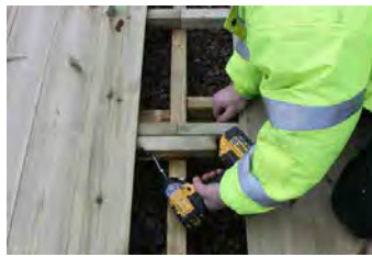
Step 2 - Ensure the panels are placed with the floor joist ends butted together, and that the joists line up. Screw together through joists.
