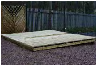
Step 1 - Ensure the shed has a level & sufficient base in place. Concrete or sleeper base is ideal. Position the floor ensuring it is level.
