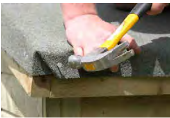
Step 23 - Fold the felt neatly at the corner and tack along the roof edge. Repeat steps 22 – 24 on the other low side.
