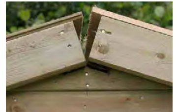
Step 12 - The two roof sections should sit down and line up as pictured. Ensure butted tight to back.
