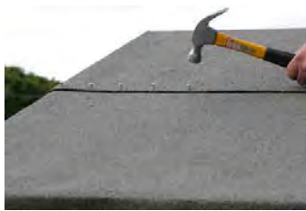
Step 24 - Now continue with the second run of felt, overlapping on top of the first.
