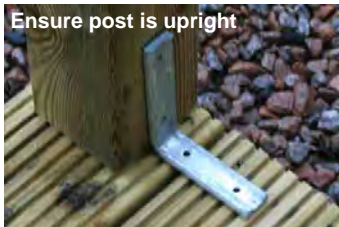
Step 18 - An 'L' shape bracket is then screwed into position at the back of each post and into the base.
