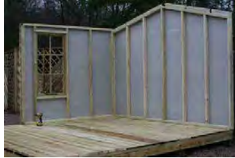
Step 6 - The second panel is positioned in place. Butted up tight to the other panel.
