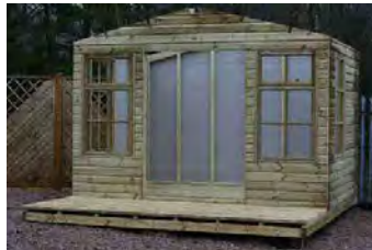
Step 10 - The last panel to be fitted and screwed into place is the front panel.
