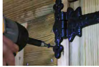
Step 29 - Fix the hinges at the top and bottom of each door using the screws provided.
