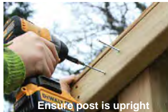
Step 19 - Use two screws through the roof framework to secure the top of the post & keep it square.
